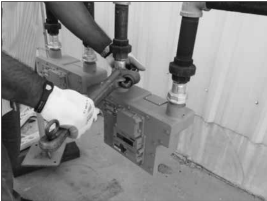
Figure 7.5 - Use a pipe wrench to tighten swivel nuts
