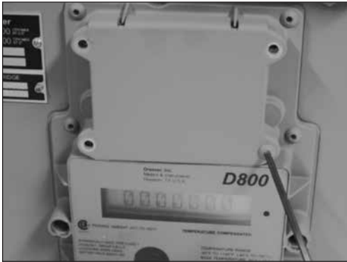
Figure 9.28 - Remove 4 screws on battery cover
