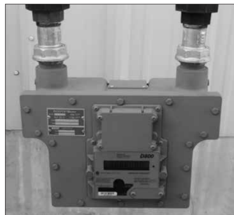
Figure 7.4 - Meter placed in line
