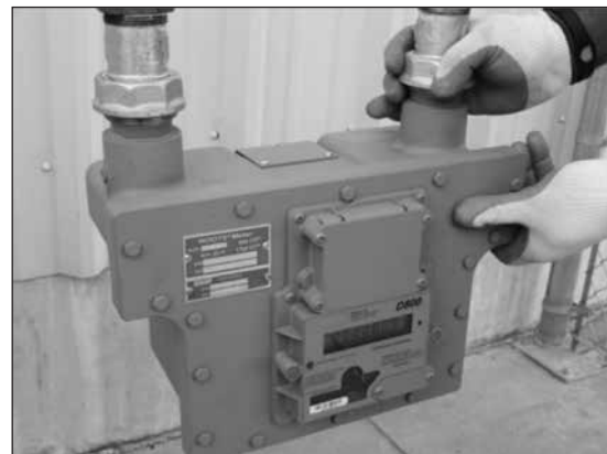
Figure 7.3 - Connect meter outlet to swivel nut on the downstream side
