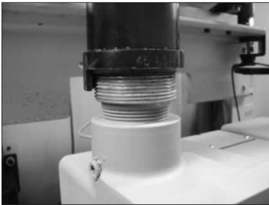
Figure 10.10 - SNAP connections properly fitted to meter
