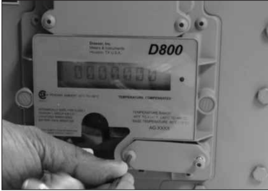
Figure 9.1 - Remove two button head screws
