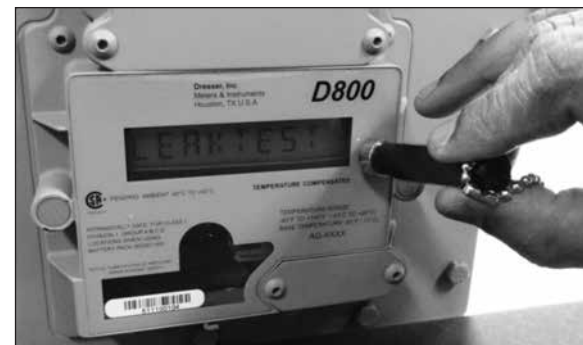
Figure 7.7 - Scroll to LEAKTEST screen
