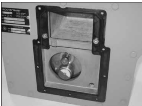
Figure 9.14 - Place gasket onto meter
